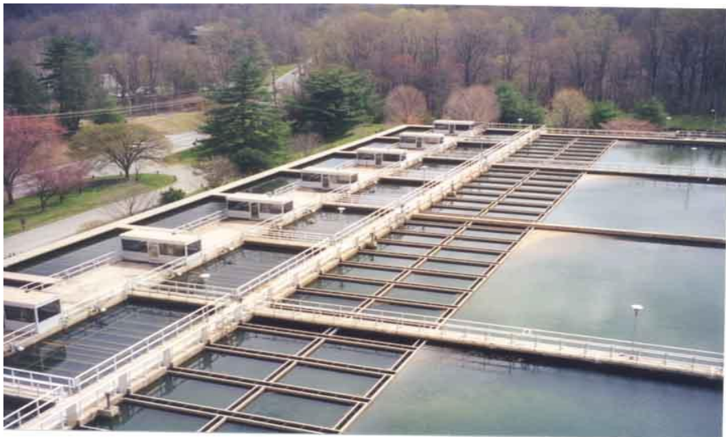
Fig: Rectangular Sedimentation Tank
